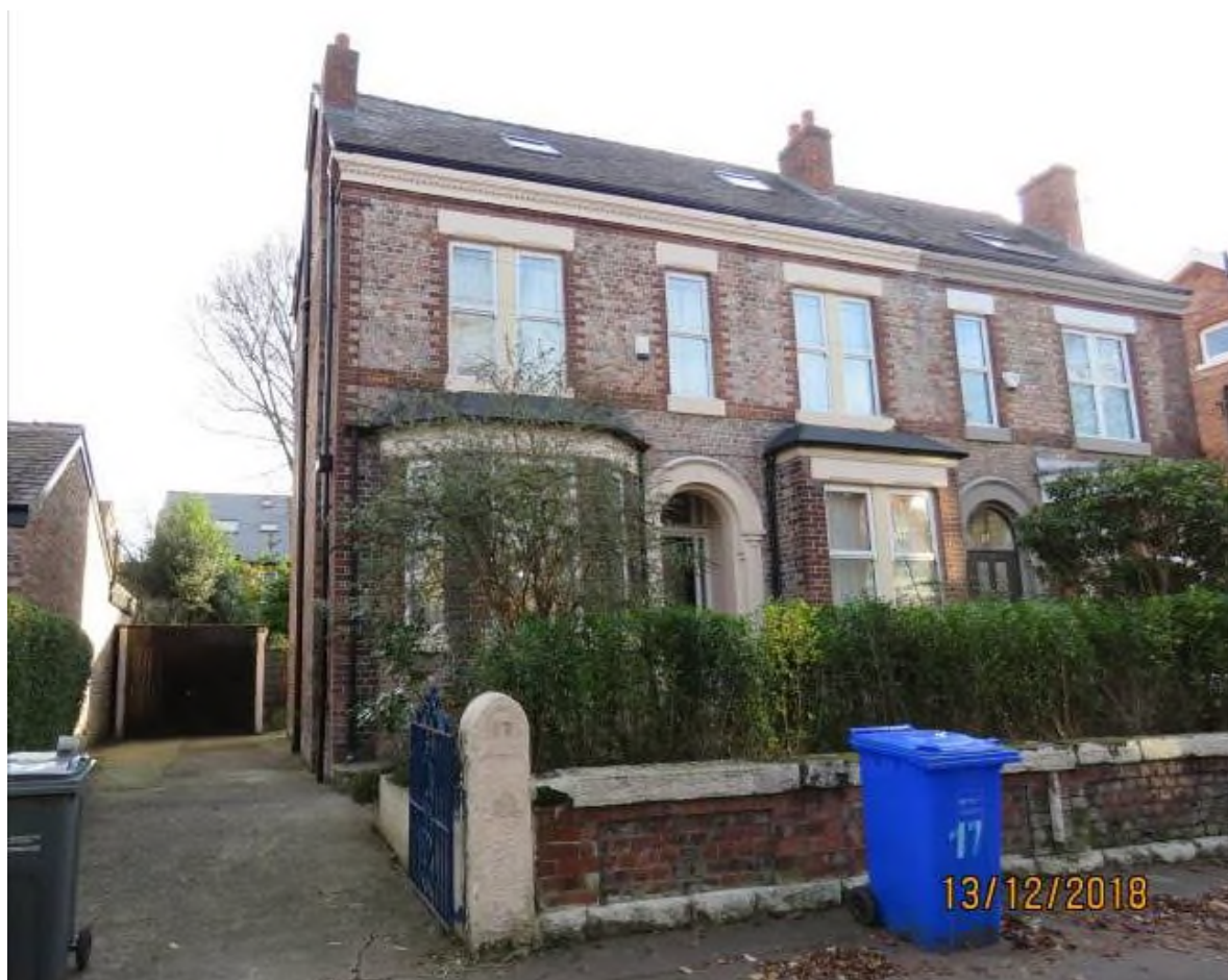
Front elevation with driveway
