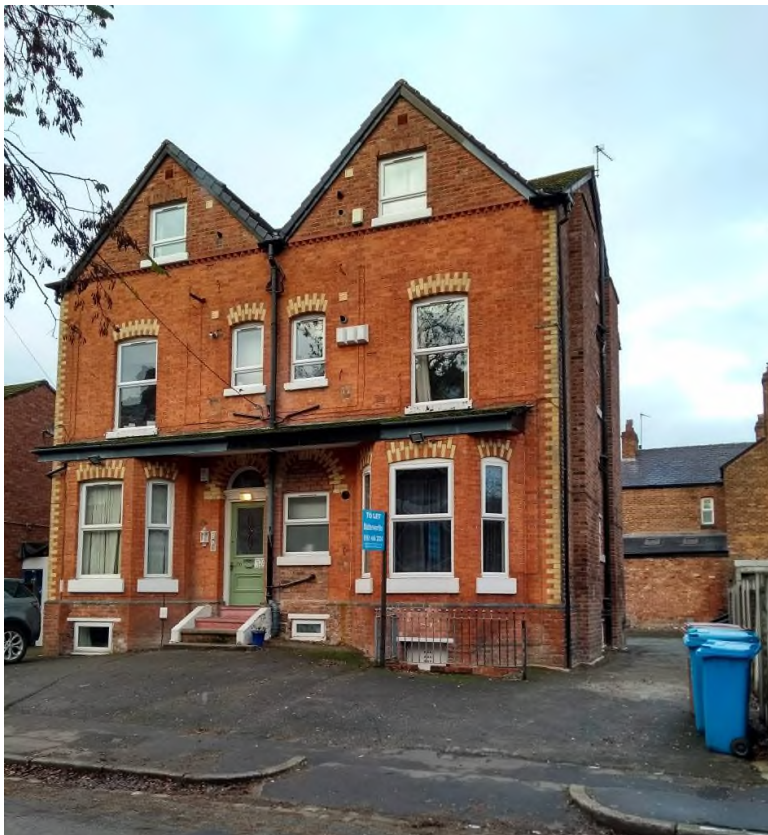
Semi's converted to flats on Northen Grove – loss of gardens and boundary walls
